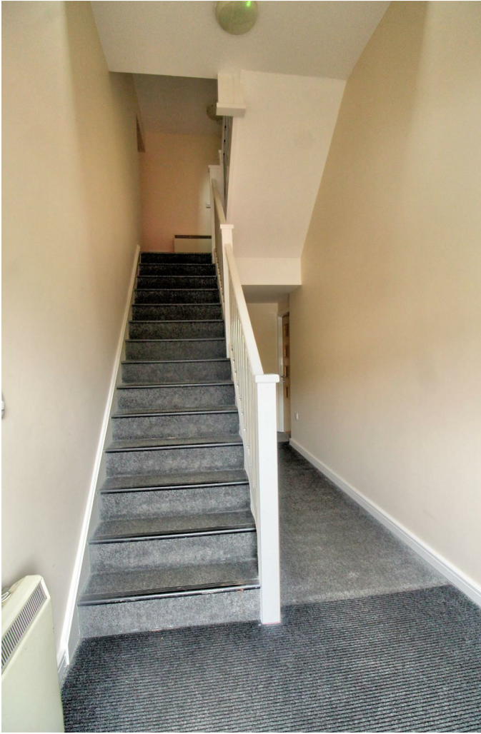
Main hallway with intercom system
